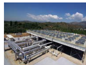
Turkey Geothermal power Dora II
